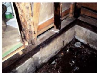
柱の腐朽
