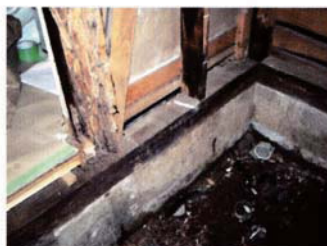
柱の腐朽
